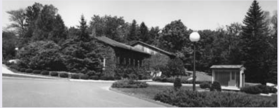
Avon's town offices, housed in former buildings of the Ensign-Bickford Fuse Company, are part of a contested National Register district nomination.
